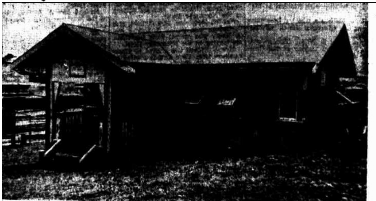
The new C.W.A. rest room at Yeppoon.
