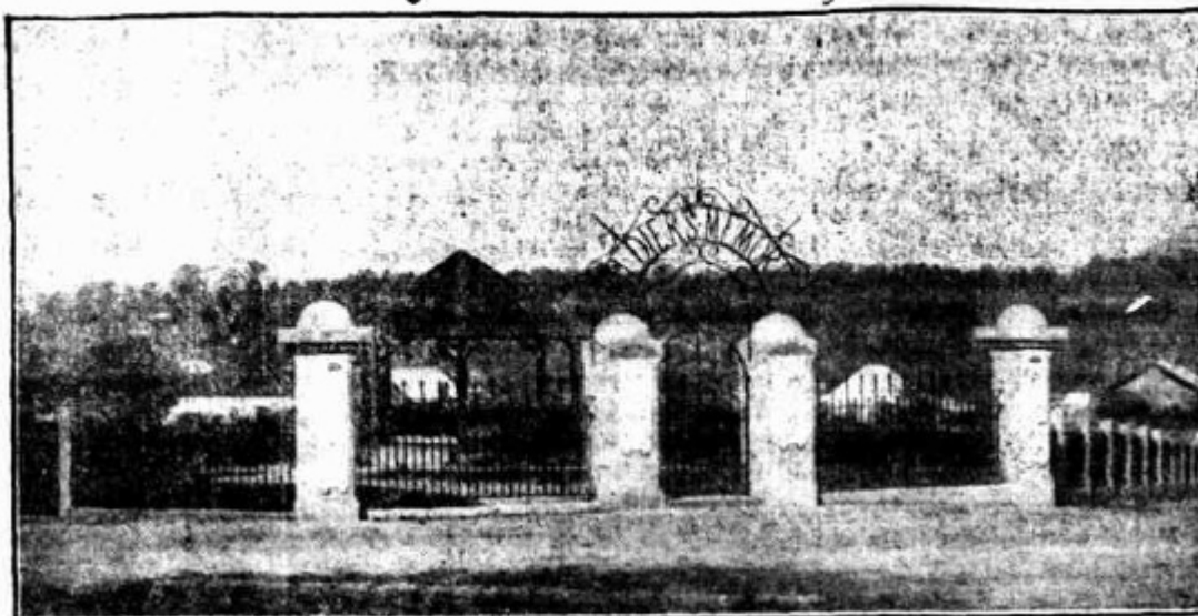
The above photo shows Tablets fixed to Pillars at main entrance to Gardens with Rotunda in background.
