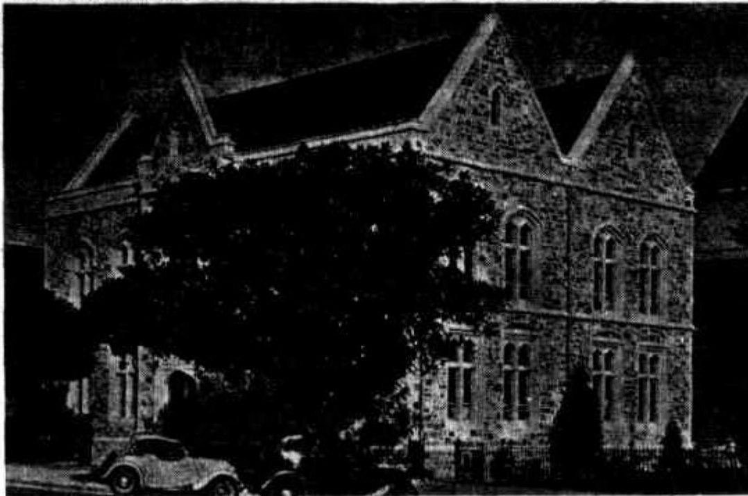
View of the New Education Building erected at eastern end of Cathedral
